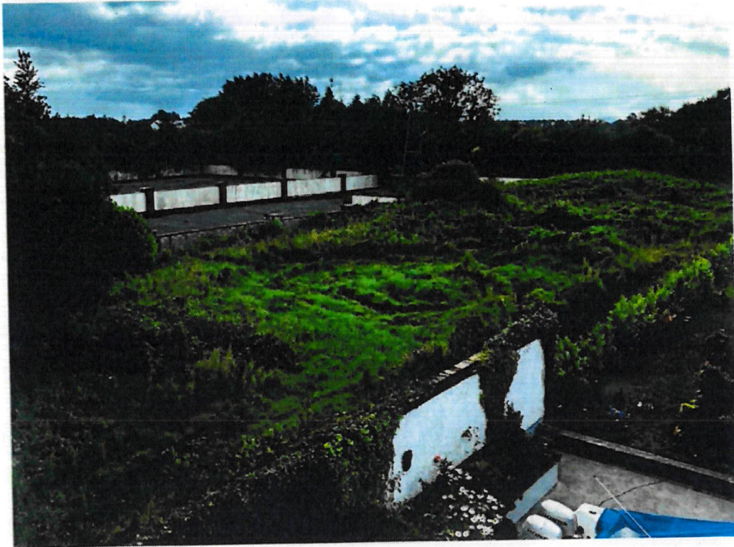
Photo 022 - Hard landscaped courtyards at the rear of D1 & D2
